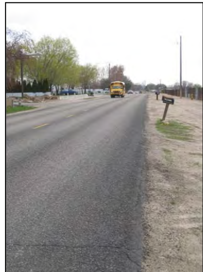
Airport Road is an existing rural road serving the Nampa Municipal Airport and provides a connection between the Ada/Canyon county line (McDermott Road) and Garrity Boulevard.
